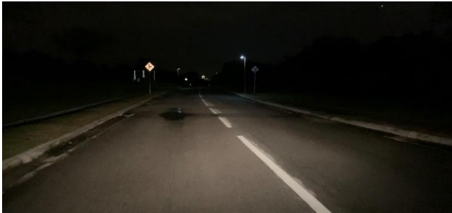
Figure 2: A representative image of the roadway in the rural setting (Wetland Park, Putrajaya).
